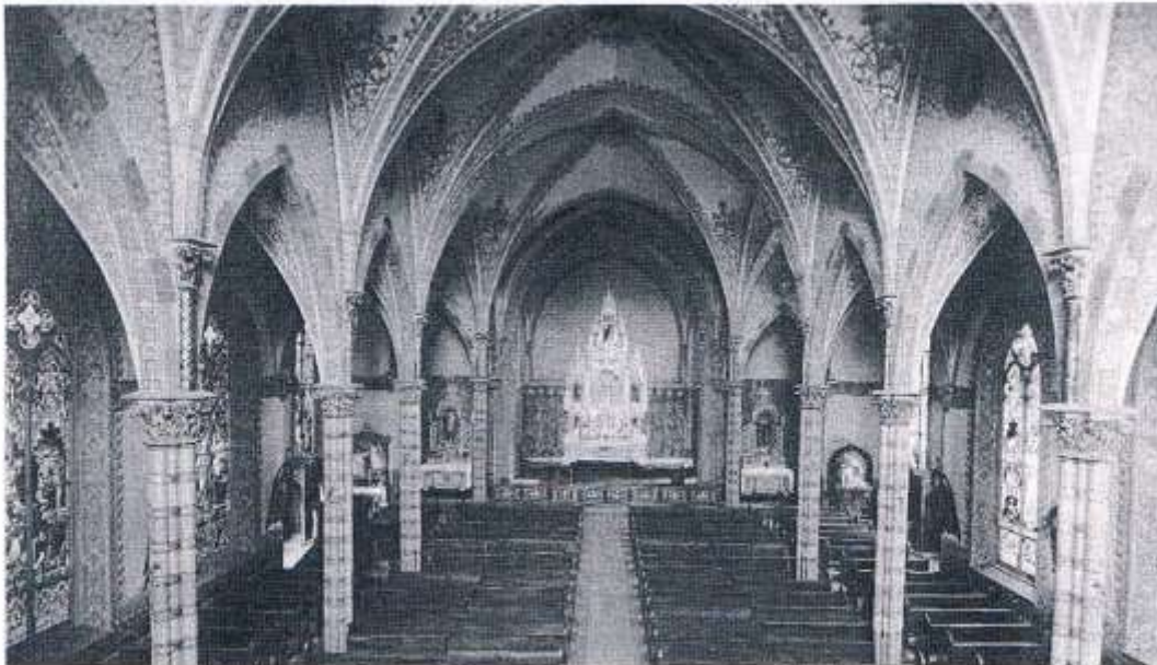
Church interior, after the 1919 frescoping, with the new main altar.
