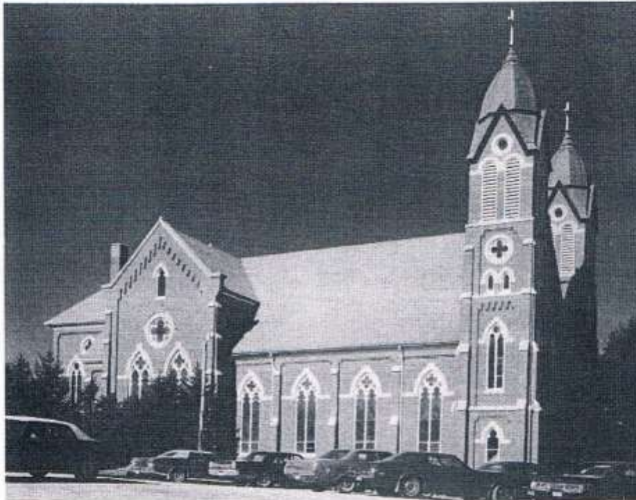
Side view of St. Luke's Church, 1977.
